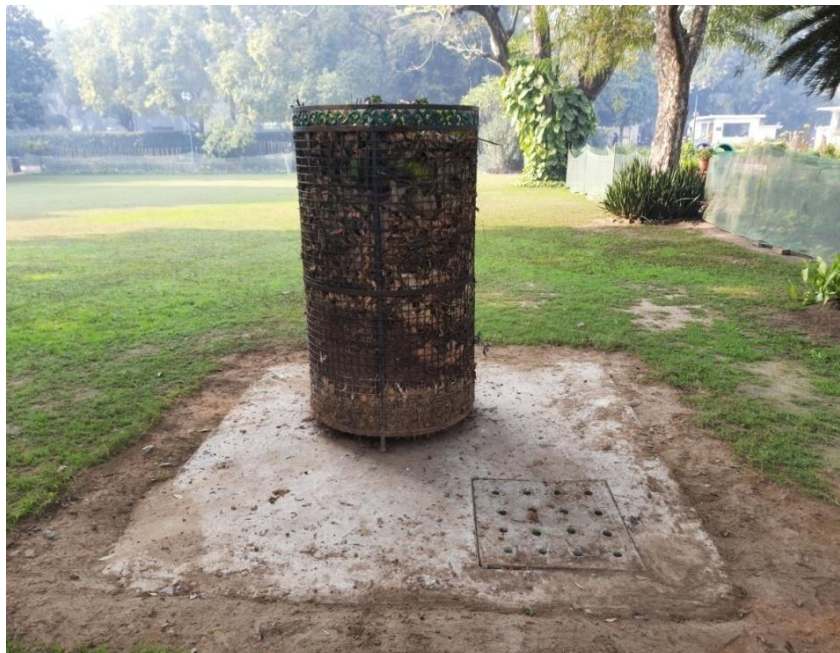
Rain Water Harvesting Pit (Total Number: 9, Additional 3 under construction)
