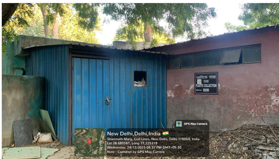
Plastic waste collection room
